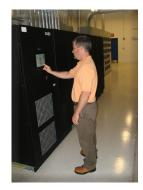
the VDC-XE units work seamlessly with energy-efficient three-phase UPS units, but take up a third of the room of comparably-sized batteries. "Space was another concern," said Ganus. "I was very limited on where I could house the power systems and three battery cabinets wouldn't fit into our equipment room." Besides a smaller footprint compared to batteries, flywheels don't need special cooling and can operate flawlessly from -4° F to 104° F.
