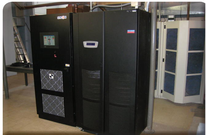
The slim footprint of the VDC flywheel is easy to pair with three-phase UPS systems.
