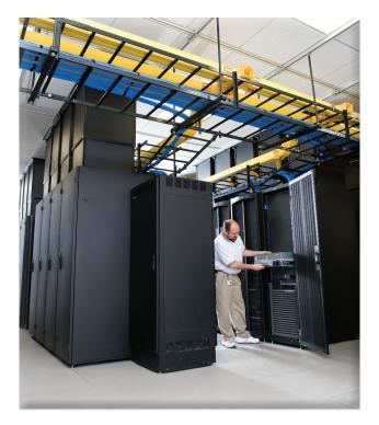
The staff also installed blanking panels and sealed floor penetrations with brush grommets. "We had several Computational Fluid Dynamic (CFD) studies done to model the data center prior to placing equipment," Briggs explained. To minimize electrical use, the data center uses occupancy/vacancy sensors on its lighting controls.
